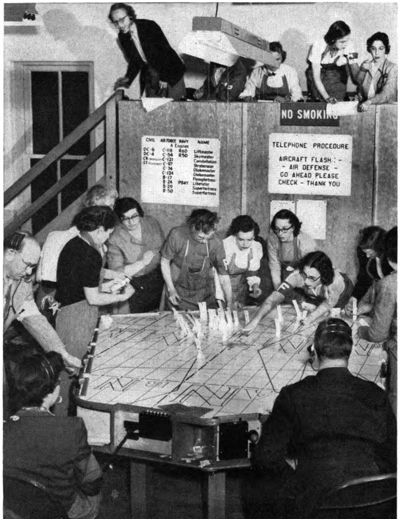
AIR RAID WARNING SYSTEM —The Bell System is providing nationwide communication facilities for defense at the request of military authorities. The photograph shows aircraft movements being mapped in a Civilian Defense "filter" center, as reports from strategic observation posts are received by telephone.
